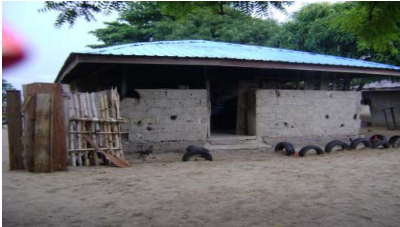
One of the many schools in Tolu school complex reflecting neglect
